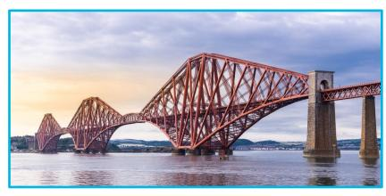
(7.6 m). Each main span comprises two 680 ft (210 m) cantilever arms supporting a central 350 ft (110 m) span girder bridge. The three great four-tower cantilever structures are 340 ft (104 m) tall, each 70 ft (21 m) diameter foot resting on a separate foundation. The southern group of foundations had to be constructed as caissons under compressed air, to a depth of 90 ft (27 m). At its peak, approximately 4,600 workers were employed in its construction.
