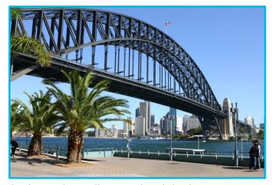
Records, it is the world's widest long-span bridge and its tallest steel arch bridge, measuring 134 metres (429.6 ft) from top to water level. It is also the fourth-longest spanning-arch bridge in the world. The arch is composed of two 28-panel arch trusses. Their heights vary from 18 m (55.8 ft) at the center of the arch to 57 m (176.7 ft) (beside the pylons).
