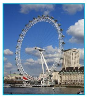
The technology employed had previously been used to erect North Sea oil rigs. The London Eye is often mistakenly called a Ferris wheel. This is not the case: first, the passenger capsules are completely enclosed and are climate controlled; secondly, the capsules are positioned on the outside of the wheel structure and are fully motorized; and third, the entire structure is supported by an A-frame on one side only.
